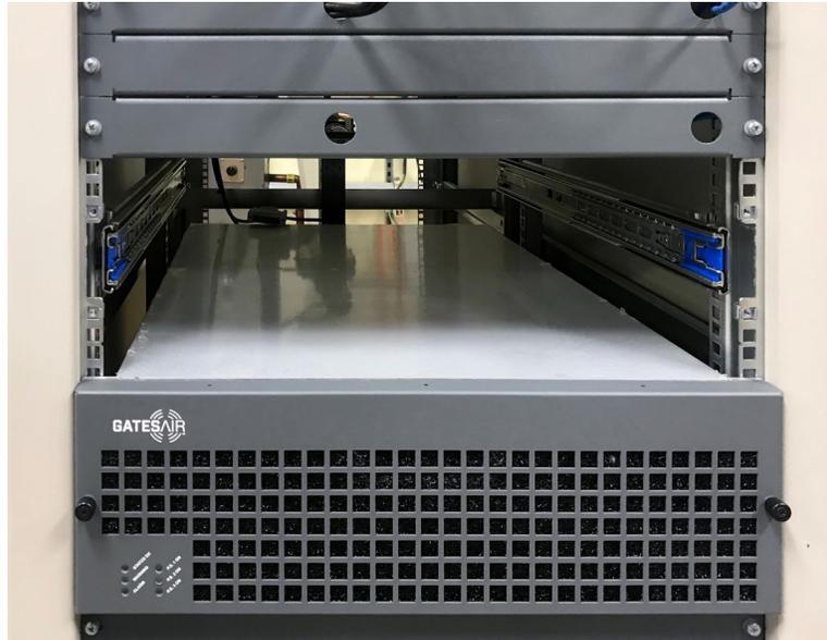
Figure 6: Sliding guides insertion
